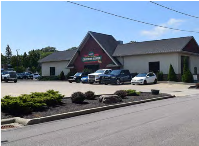
Auto Collision Center located at the intersection of South Court Street and Mill Street.
