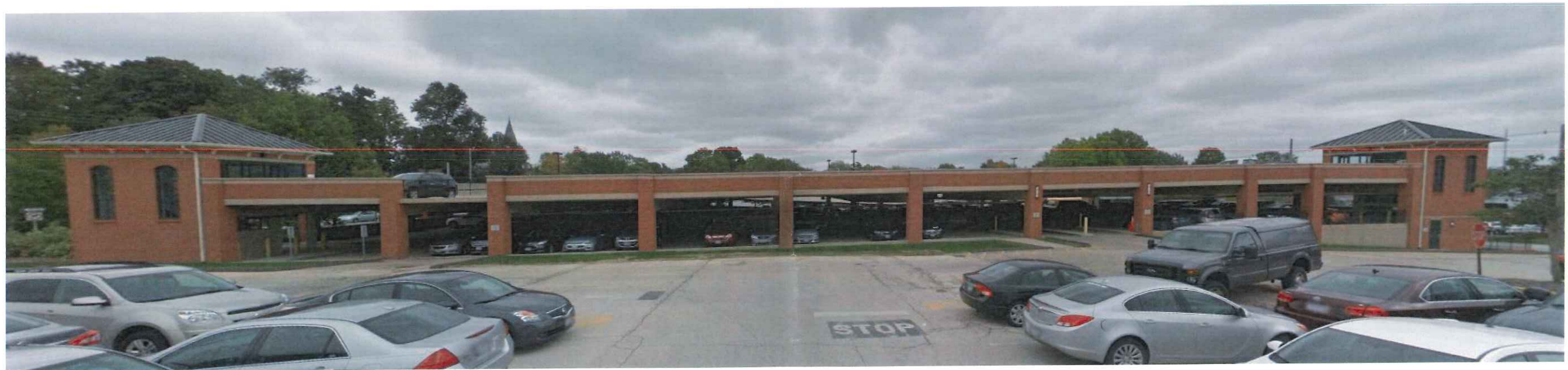
Parking Garage - West Side
